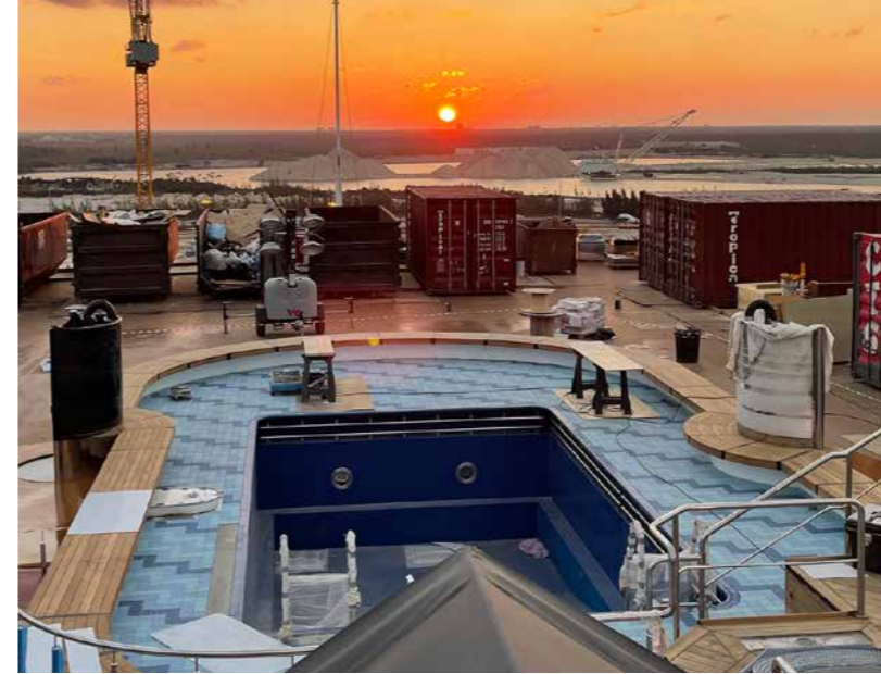
Aft pool refit
