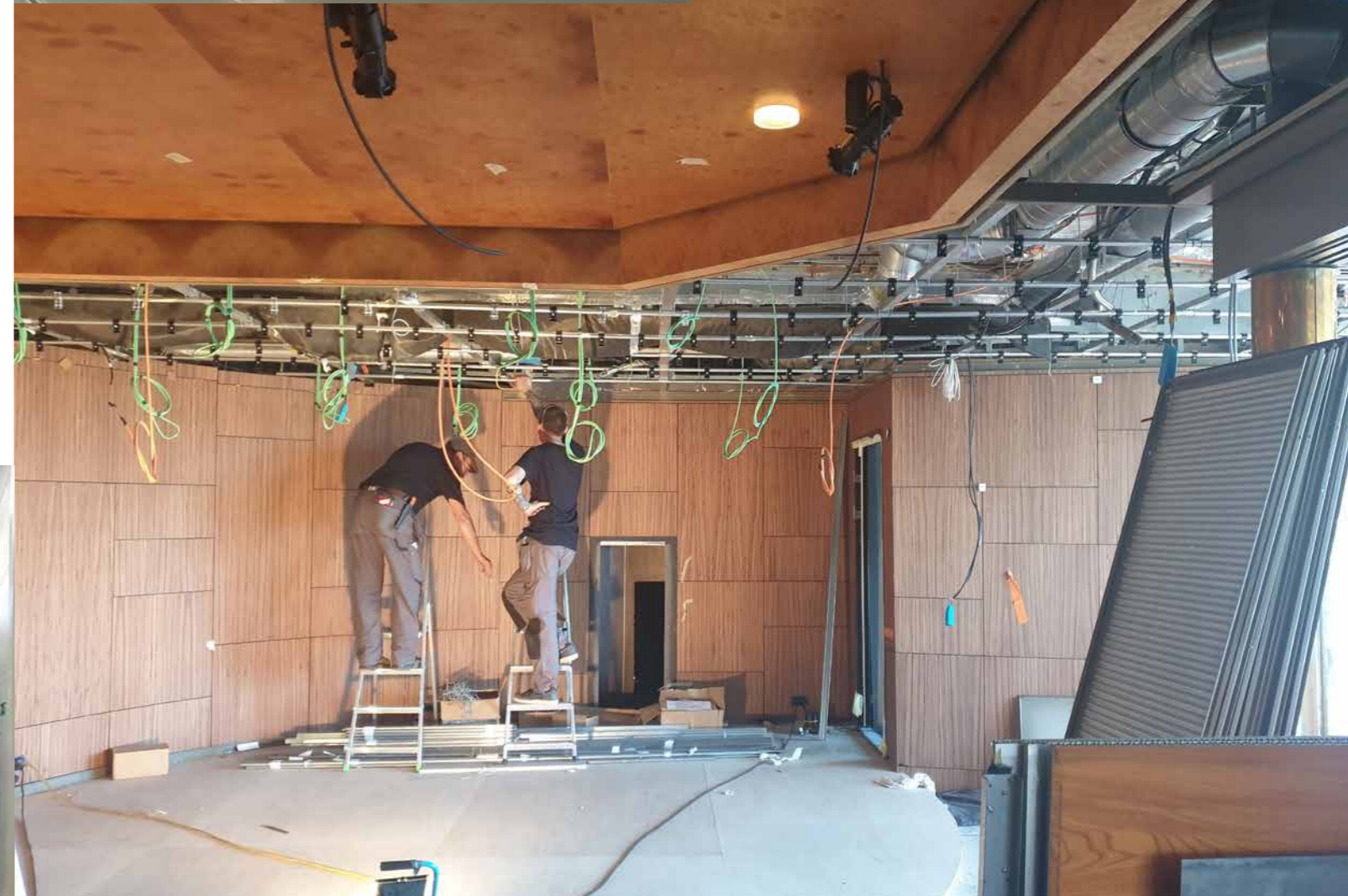
Panels Installation - Lincoln Center Stage - Holland America Line
