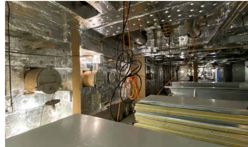
Insulation Installation - Newbuilding - Willem van Rubroek
